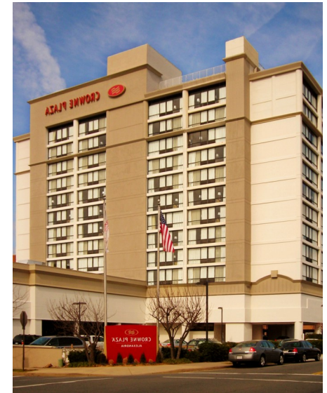
The newly renovated Crowne Plaza Old Town Alexandria
